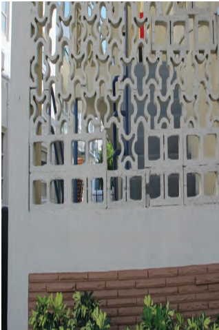
REPAIRS USING INCORRECT MATERIALS
