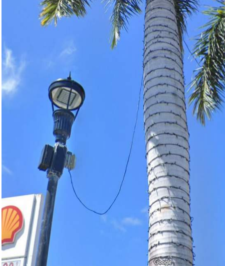
UNSAFE WIRING
