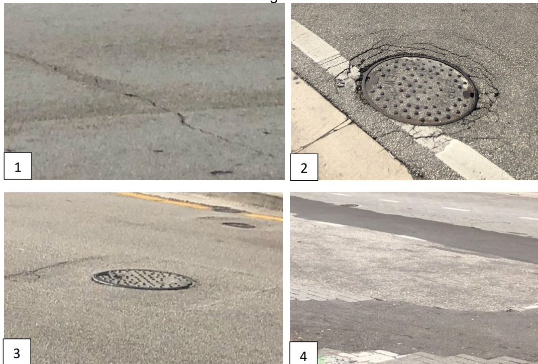
Figure 2-1 EXISTING PAVEMENT CONDITION (1-2. CRACKING, 3. DEPRESSION, 4. UTILITY CUT)
