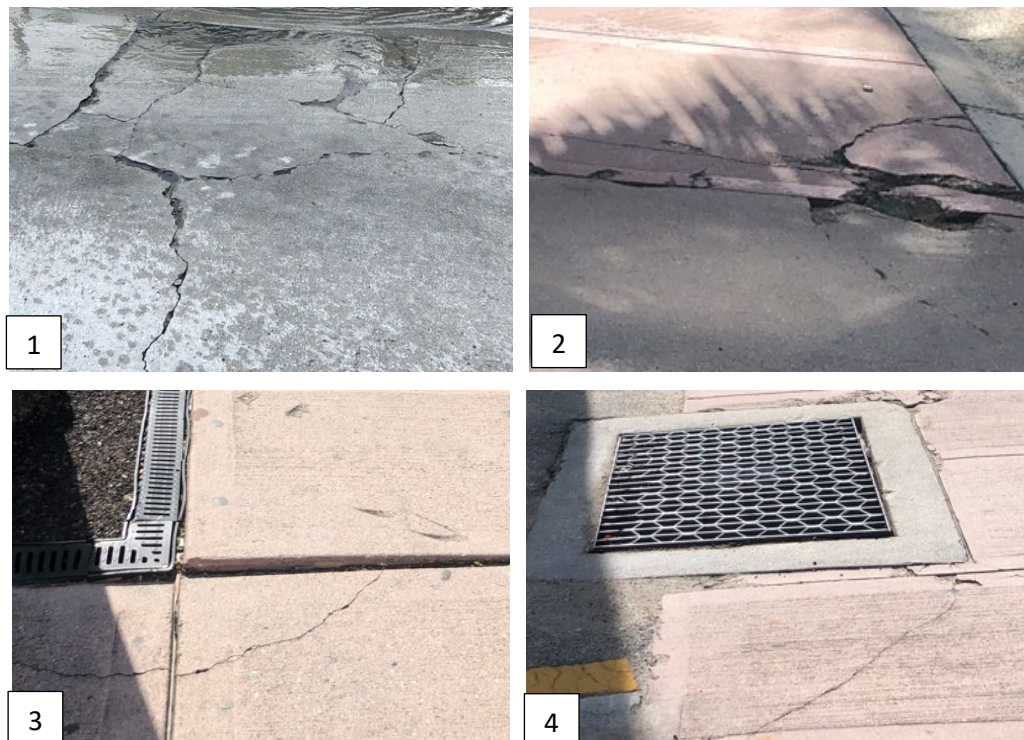
Figure 2-2 SIDEWALK DEFICIENCIES (1-2. CRACKING, 3. TRIP HAZARD, 4. NON-ADA GRATE)
