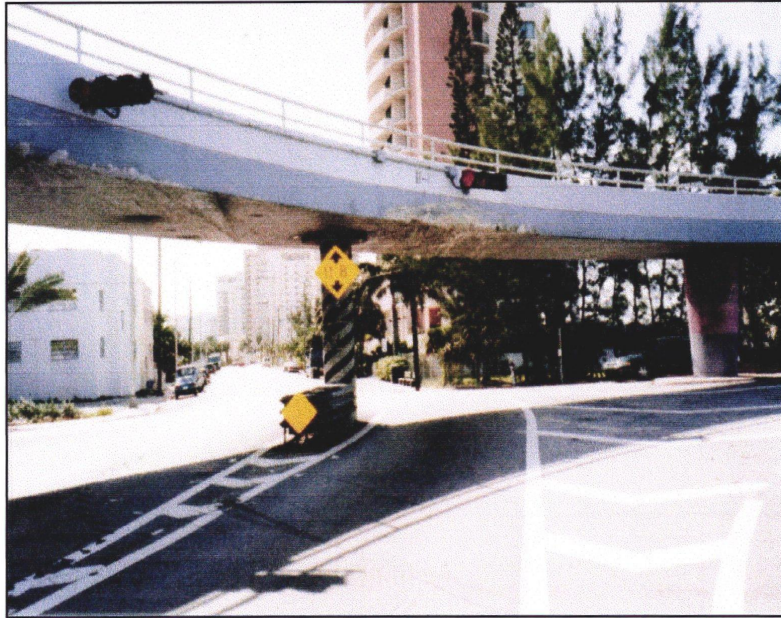
Figure 5. 63rd Street Flyover - Southbound on Indian Creek Drive denoting vehicle impacts on the flyover.
