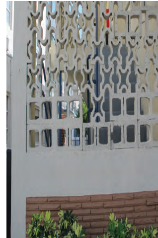
REPAIRS USING INCORRECT MATERIALS
