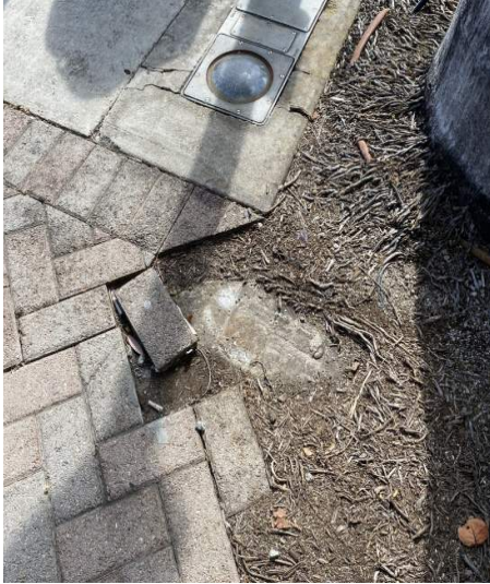
LOOSE CONCRETE PAVER
