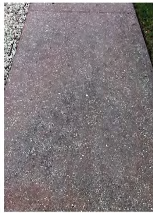
INTEGRAL COLOR RED CONCRETE WITH EXPOSED SHELL AGGREGATE
