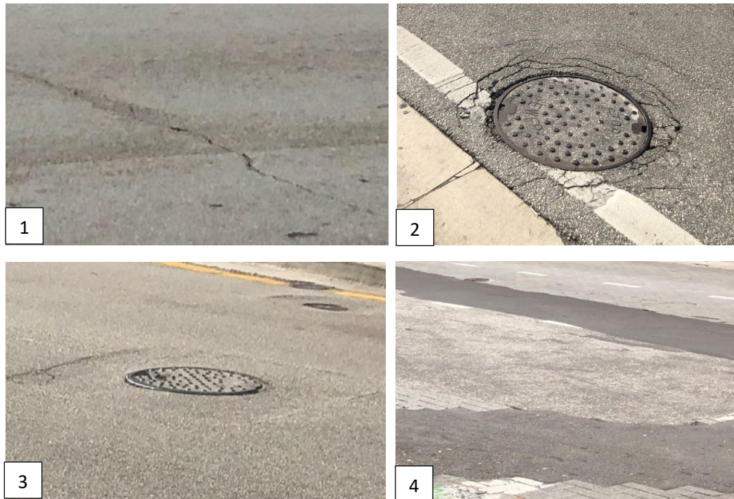
Figure 2-1 EXISTING PAVEMENT CONDITION (1-2. CRACKING, 3. DEPRESSION, 4. UTILITY CUT)
