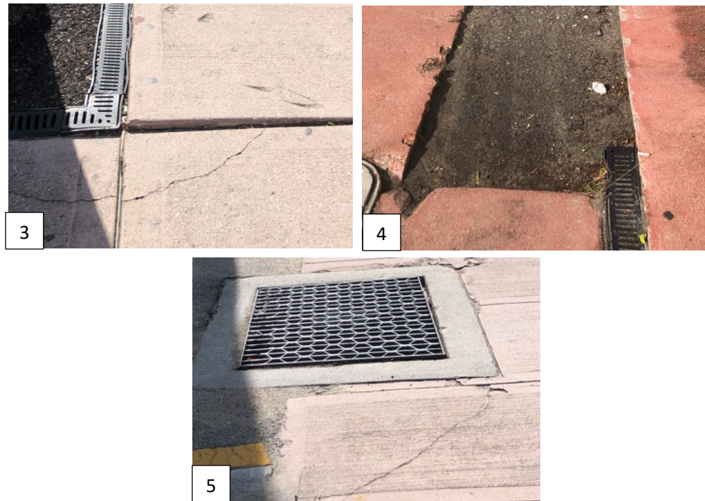
Figure 2-2 SIDEWALK DEFICIENCIES (1-2. CRACKING, 3-4. TRIP HAZARD, 5. NON-ADA GRATE)
