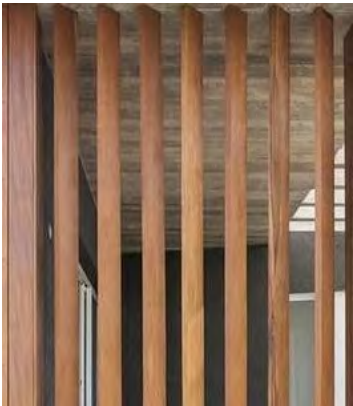
ARCHITECTURAL ALUMINUM LOUVERS WITH WOOD FINISH
