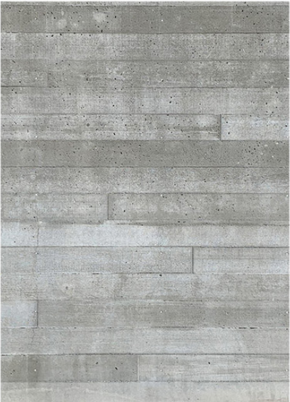
7. ARCHITECTURAL FEATURE WALL BOARD FORMED CONCRETE
