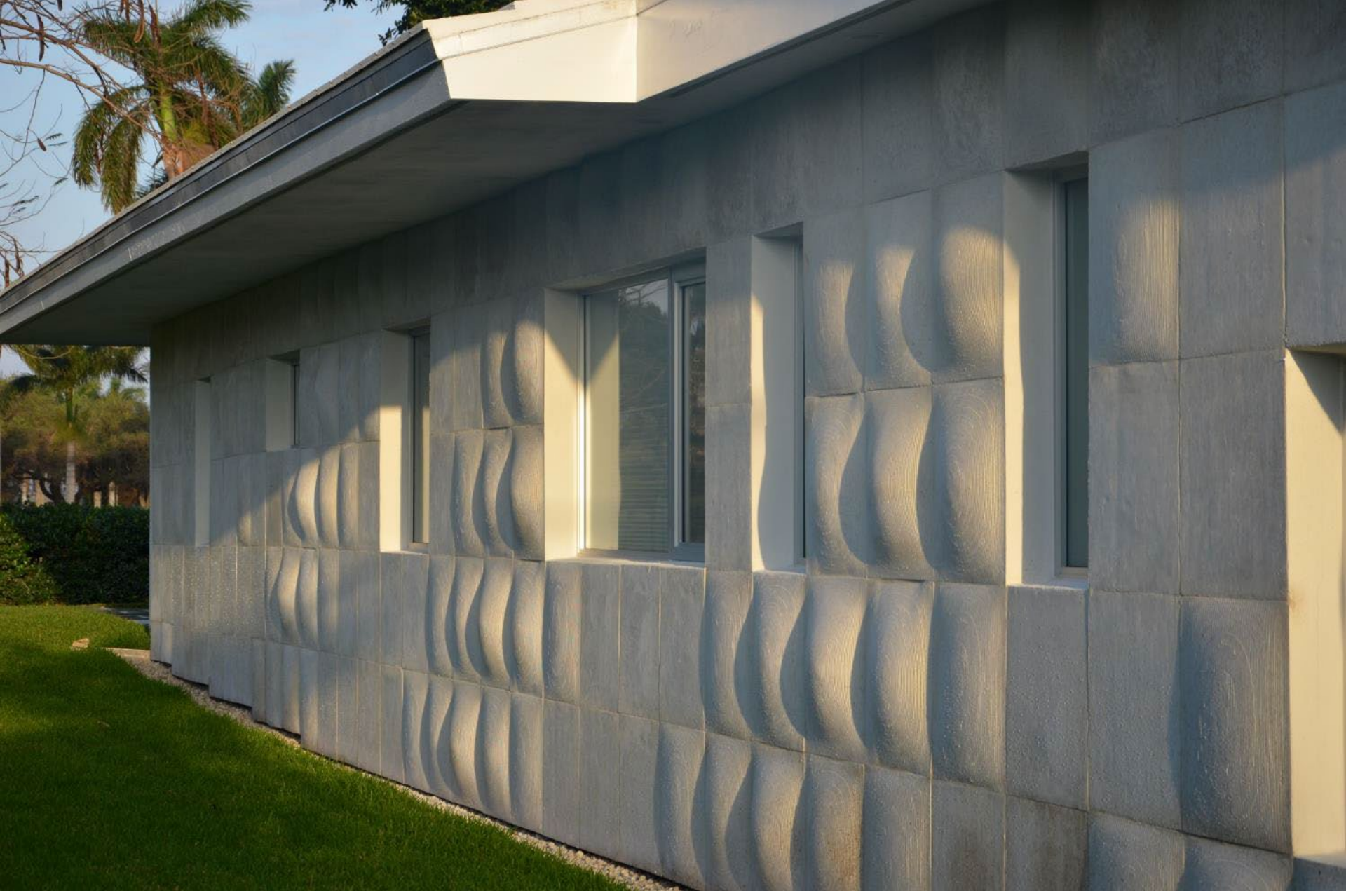
The overall pattern consisted of four unique tiles, each bulging incrementally, arranged into a playful diagonal wave pattern on the exterior. Towards the back of the site, the tiles were trimmed to step up as the grade increase for site drainage.
