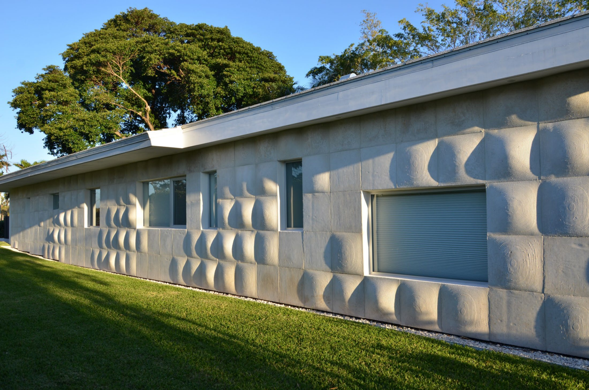
The south facing façade, which absorbs most of the solar exposure throughout the day, is clad with the unique material, insulating the interior.
