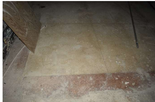
Figure 266. Detail of terrazzo flooring in Room 6, August 2022.
