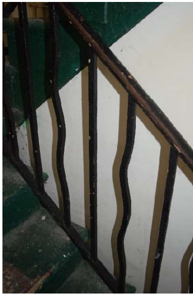
Figure 232. Detail of curved and straight balusters at front stairs, August 2022.
