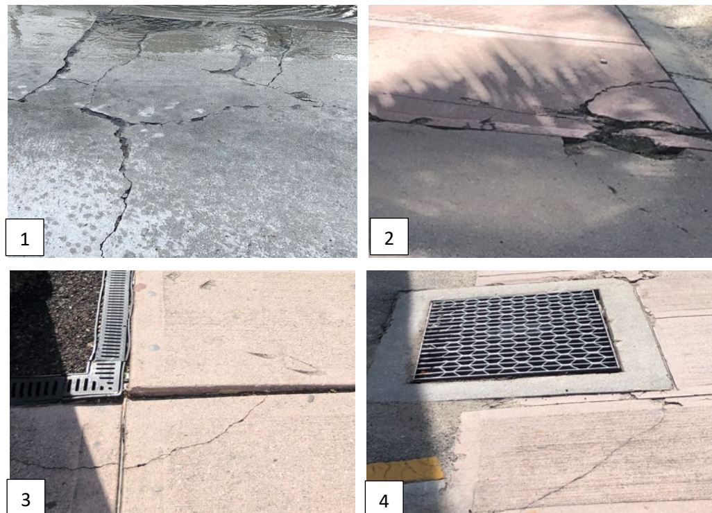
Figure 2-2 SIDEWALK DEFICIENCIES (1-2. CRACKING, 3. TRIP HAZARD, 4. NON-ADA GRATE)
