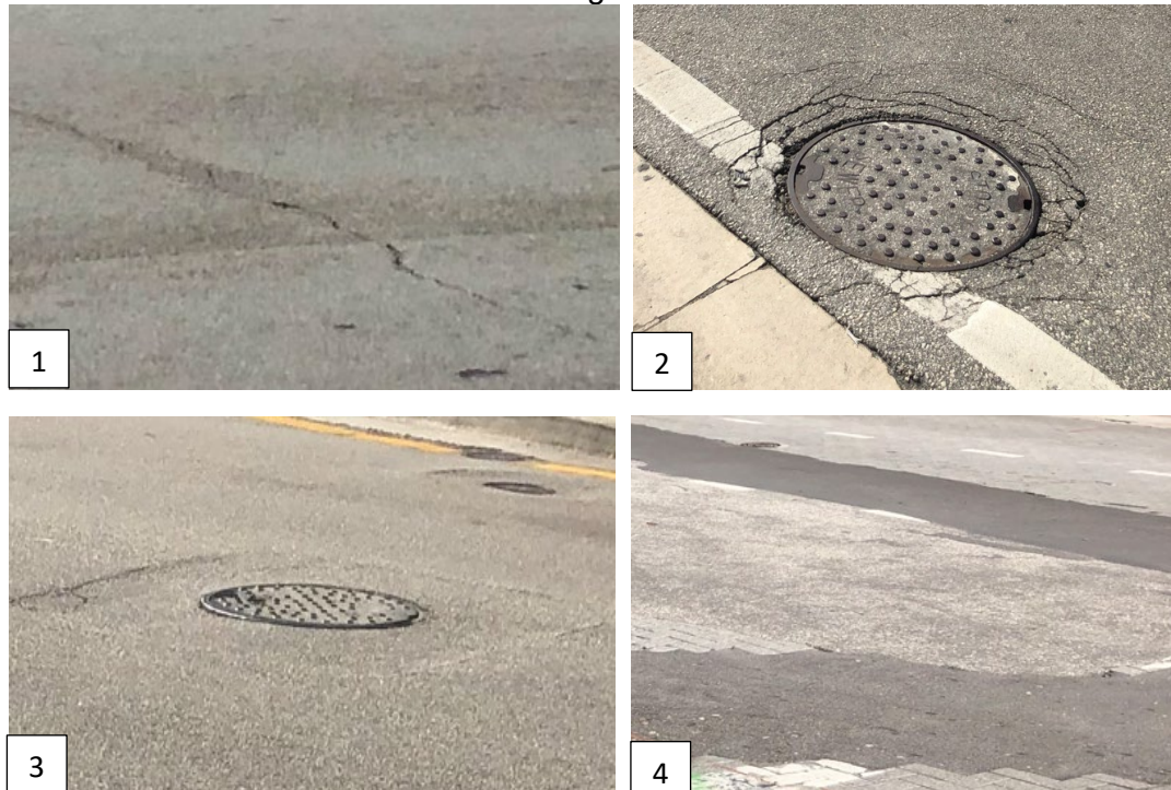
Figure 2-1 EXISTING PAVEMENT CONDITION (1-2. CRACKING, 3. DEPRESSION, 4. UTILITY CUT)
