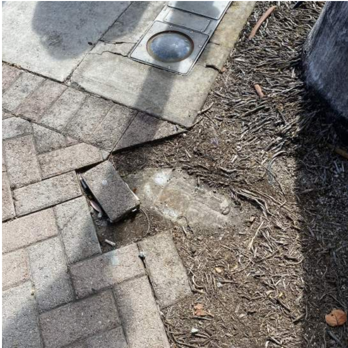
LOOSE CONCRETE PAVER
