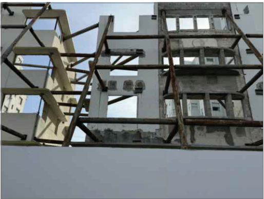
PHOTO #1-EXTERIOR SHORING N.T.S
