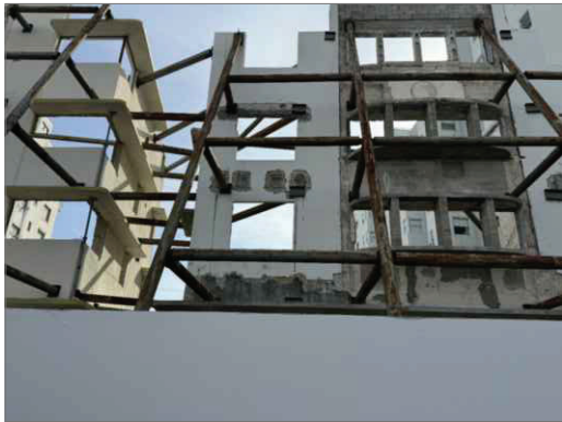
PHOTO #1-EXTERIOR SHORING N.T.S
