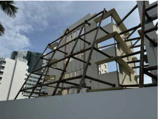
PHOTO #2- EXTERIOR SHORING N.T.S
