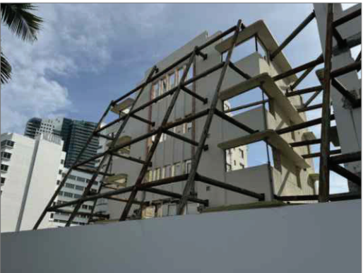
PHOTO #2- EXTERIOR SHORING N.T.S
