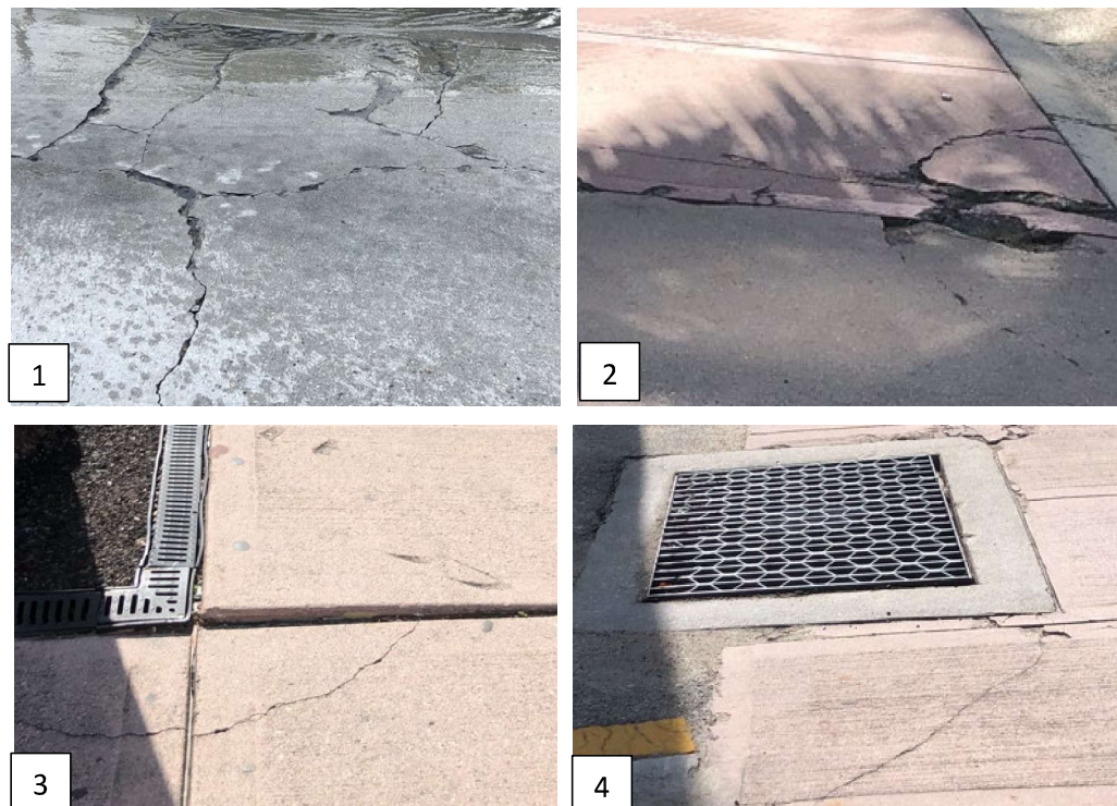
Figure 2-2 SIDEWALK DEFICIENCIES (1-2. CRACKING, 3. TRIP HAZARD, 4. NON-ADA GRATE)
