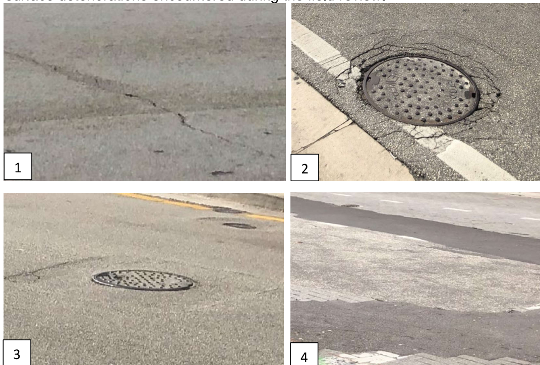
Figure 2-1 EXISTING PAVEMENT CONDITION (1-2. CRACKING, 3. DEPRESSION, 4. UTILITY CUT)
