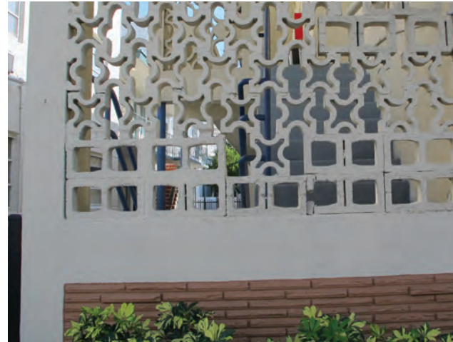
REPAIRS USING INCORRECT MATERIALS
