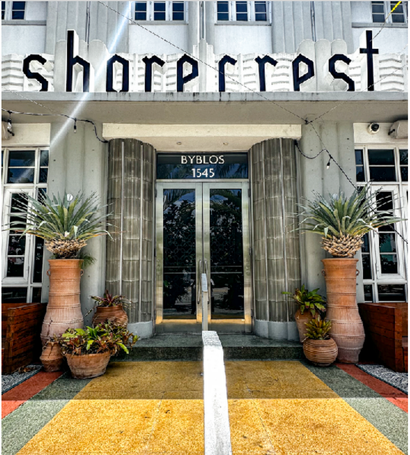
FRONT (WEST) ELEVATION FROM COLLINS AVENUE (8) SHOWING GLASS BLOCK COLUMNS ADJACENT TO FRONT ENTRANCE DOORS AND THE WAVE LIKE DETAILING BEHIND THE 'SHORECREST' SIGNAGE . THE FORMER HOTEL LOBBY IS NOW A NIGHTCLUB.(8)
