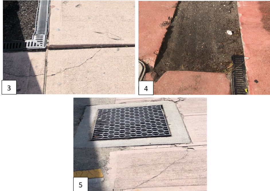
Figure 2-2 SIDEWALK DEFICIENCIES (1-2. CRACKING, 3-4. TRIP HAZARD, 5. NON-ADA GRATE)
