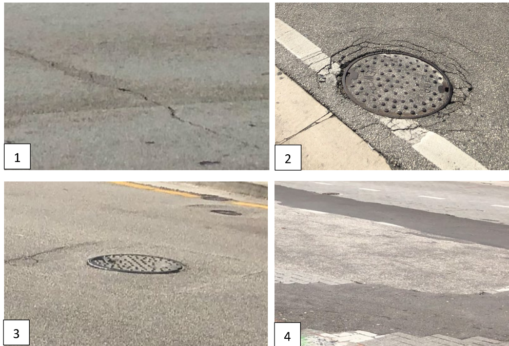
Figure 2-1 EXISTING PAVEMENT CONDITION (1-2. CRACKING, 3. DEPRESSION, 4. UTILITY CUT)
