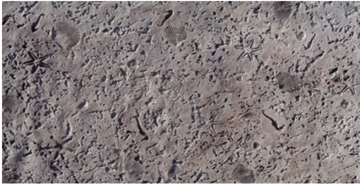
STAMPED CONCRETE SIDEWALK
