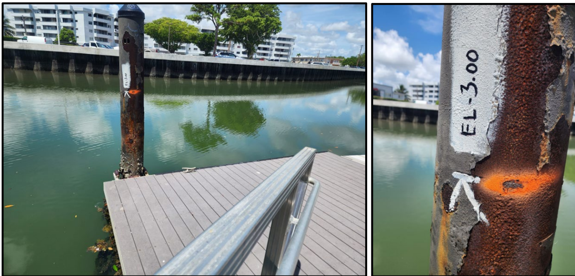
Figure III.1: Benchmark established at the Kayak Launch of the PVC showing the elevation as 3.00 feet NAVD88. Benchmark and photos courtesy of M.G. Vera and Associates and TYLin.
