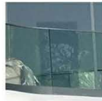
GL2 IMPACT GLASS HANDRAIL - CLEAR, RADIUSED CORNERS
