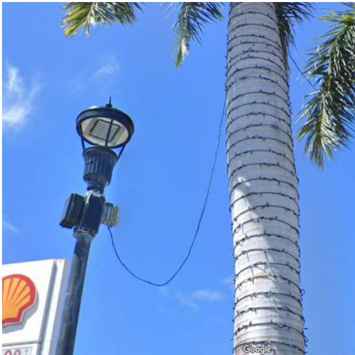
UNSAFE WIRING
