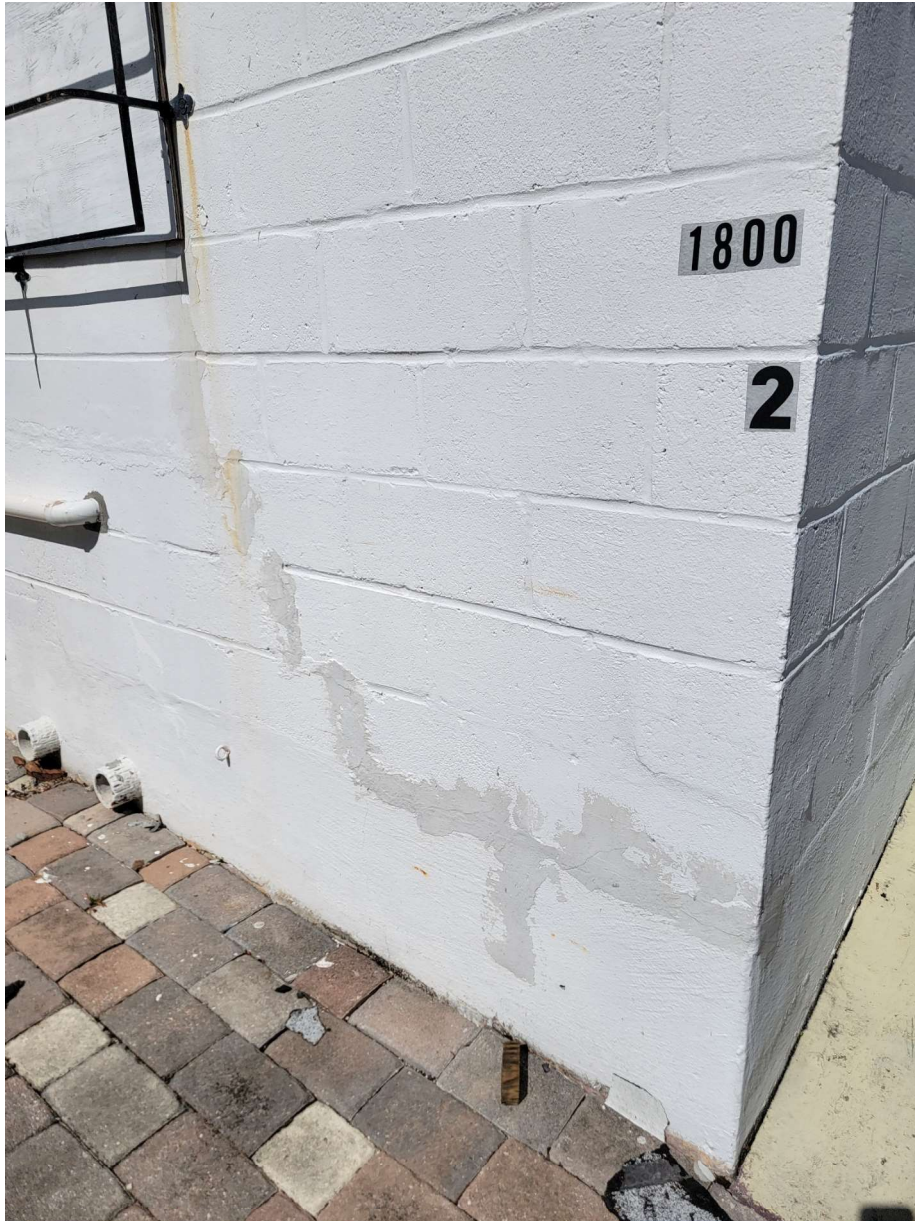
Cracks noted leading to foundations
