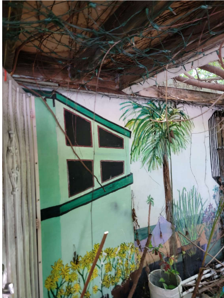
Failures noted in the exterior wood canopy
