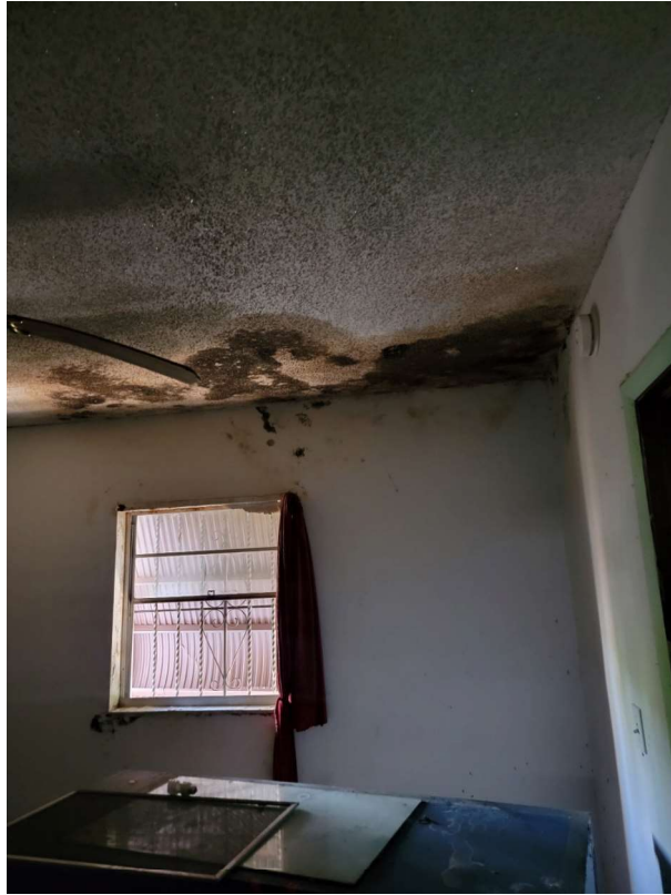
Mold is present on the interior finishes
