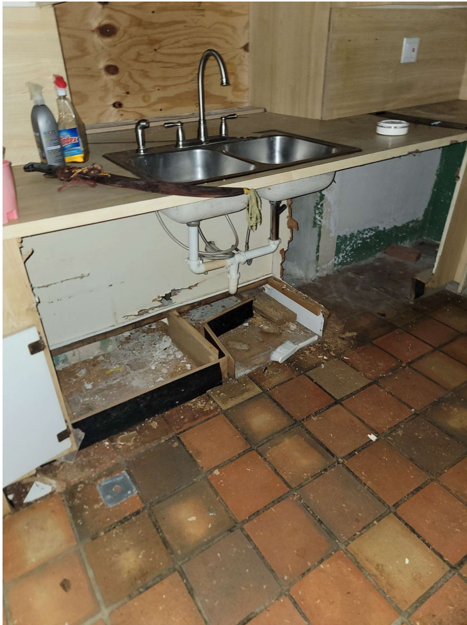
Water intrusion damages noted
