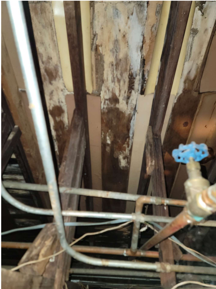
Water intrusion noticed coming from roof
