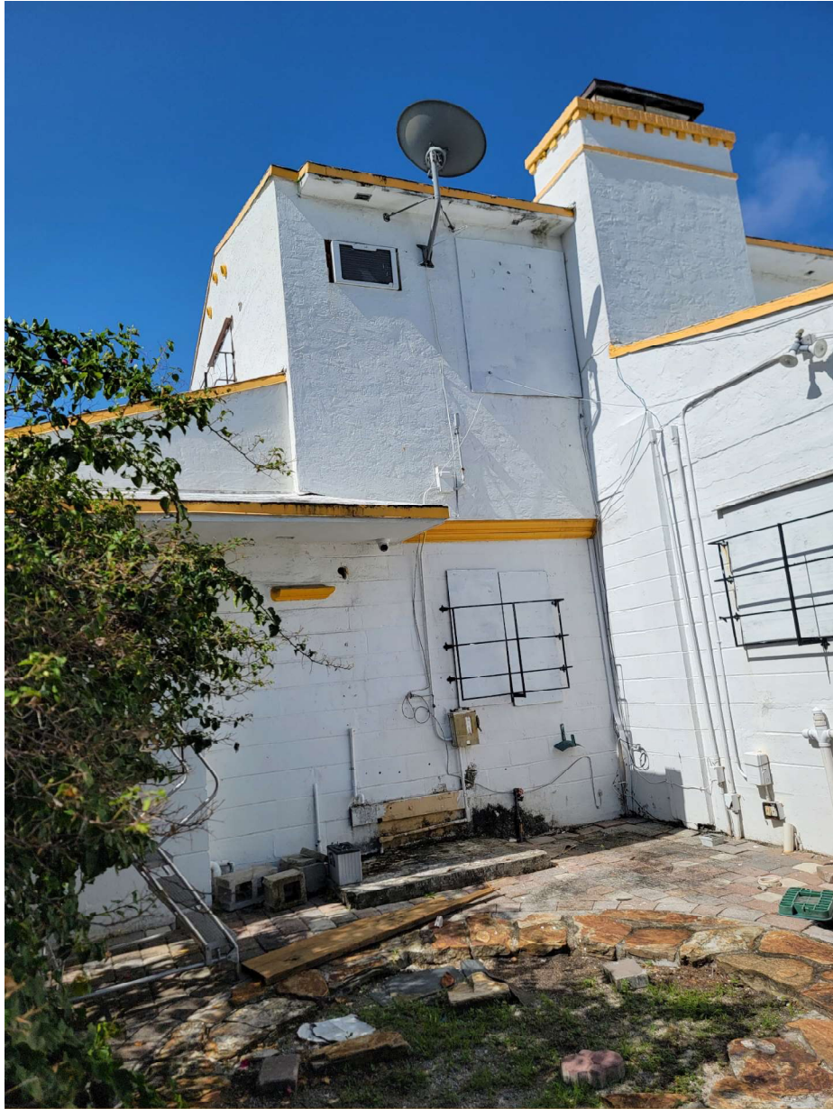
Spall and delaminated stucco present
