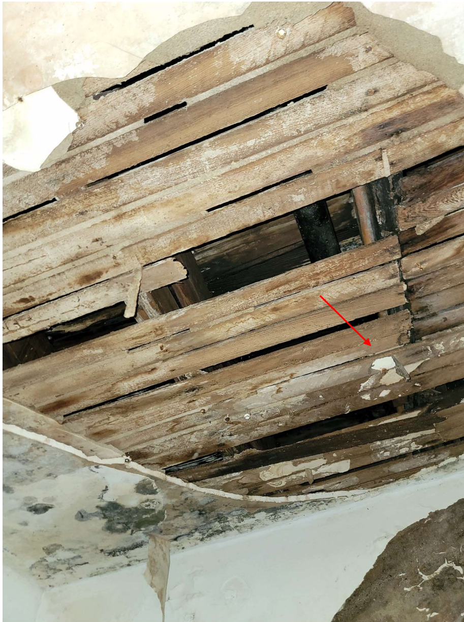
Rotted wood is noticed on the wood joist that make up the second floor of the property
