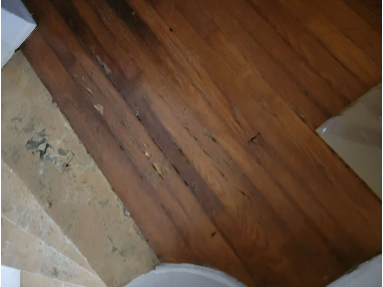
Termite damages noticed on wood floors
