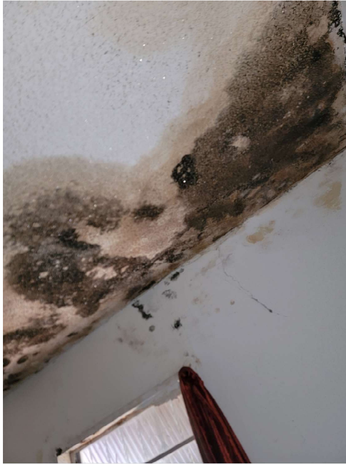
Mold and water intrusion is present
