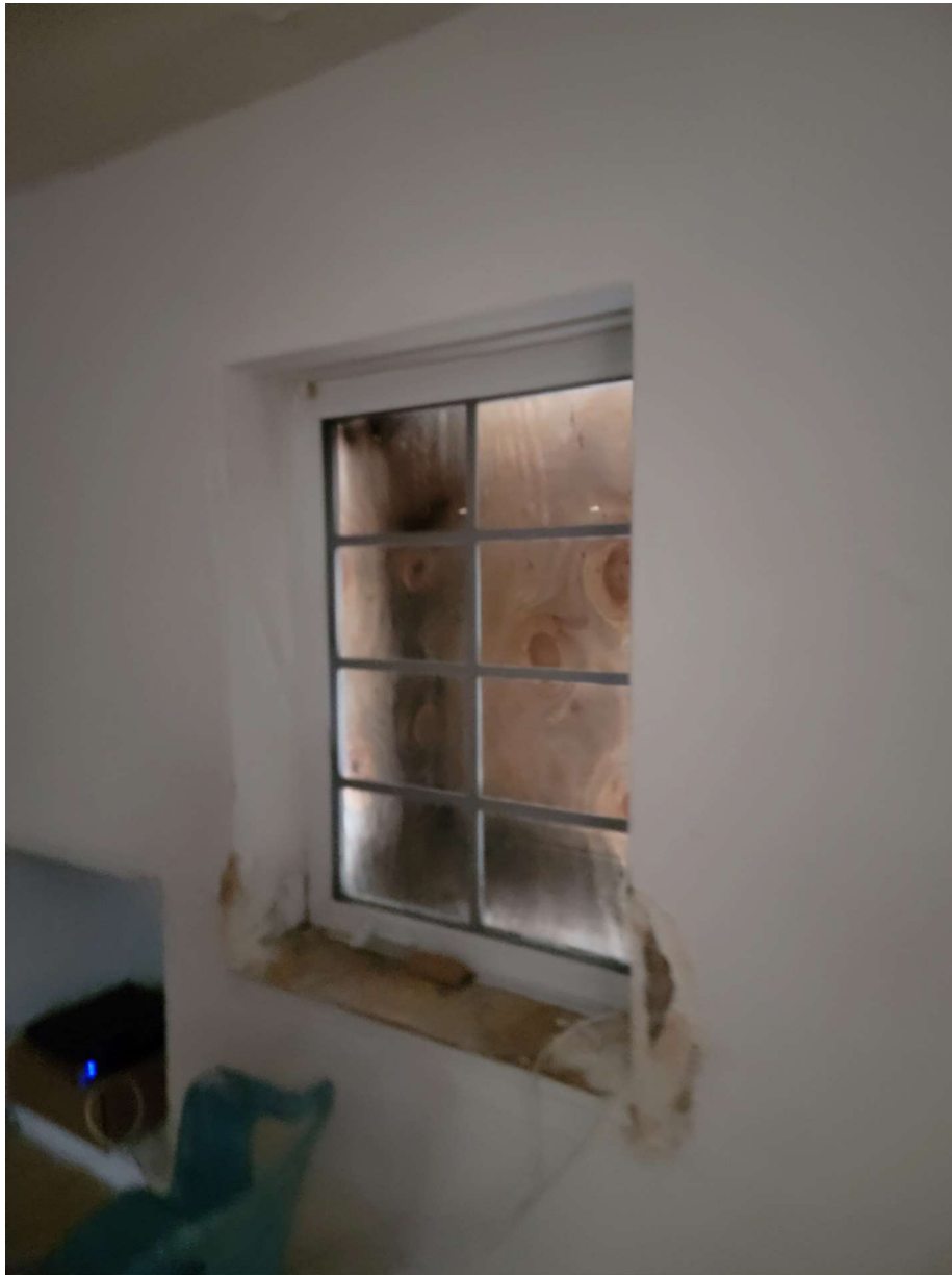
Water intrusion thru windows
