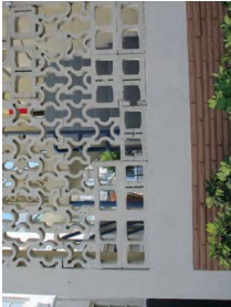
REPAIRS USING INCORRECT MATERIALS
