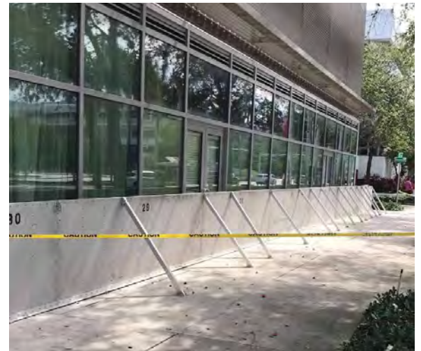
Use of flood barriers to protect building from flood damage on Pennsylvania Ave. Miami Beach. Source: Miami Beach
