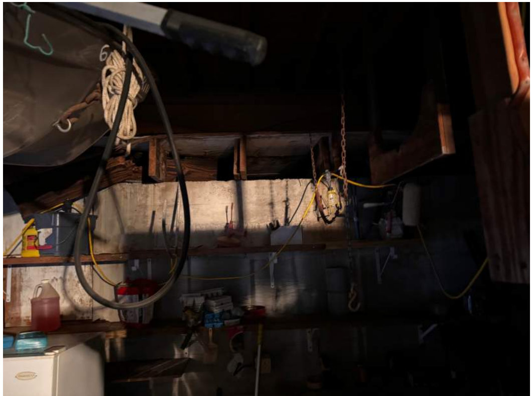
Unpermitted and non-compliant work, unstrapped and no connection
