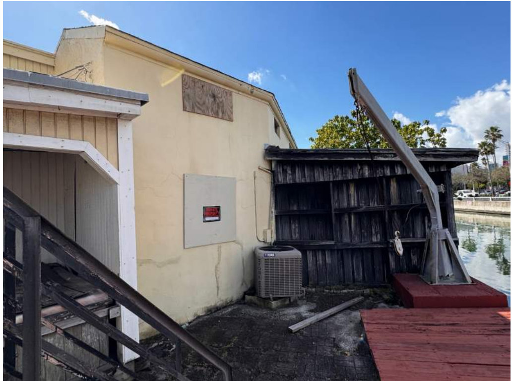
Stucco cracking, shed deterioration and dock failure
