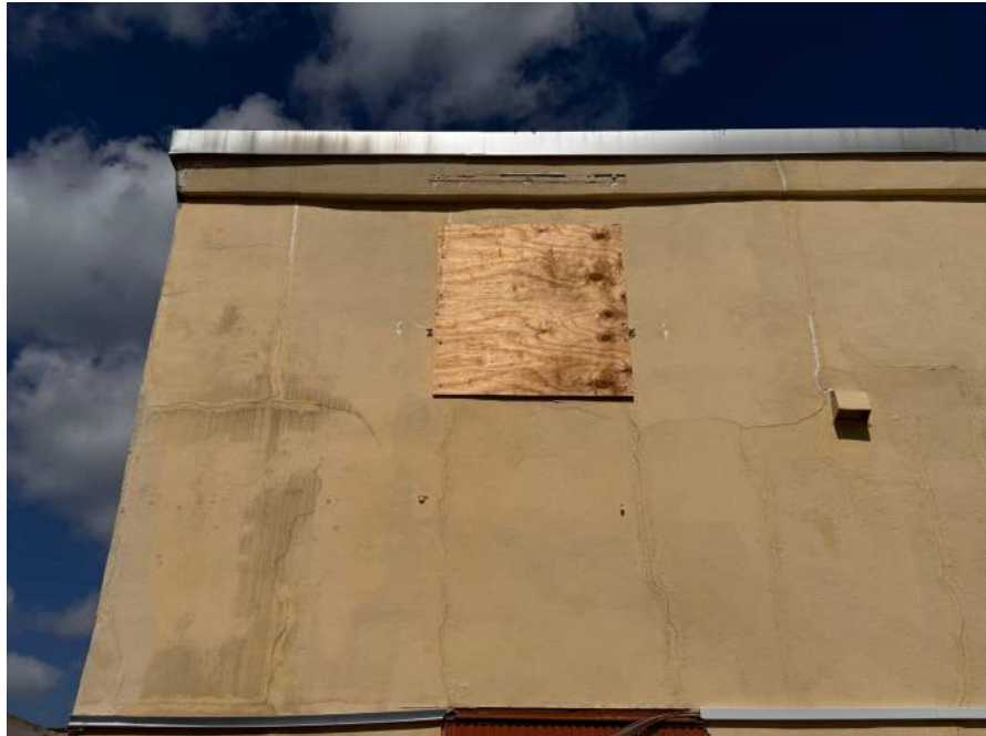
Stucco cracking throughout property
