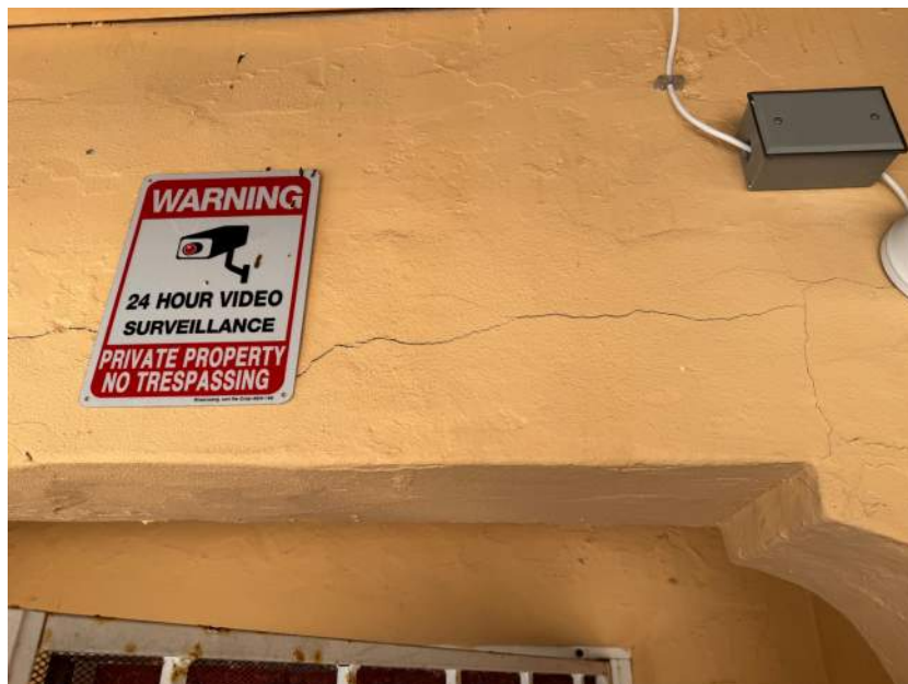
Concrete Cracking at the entrance
