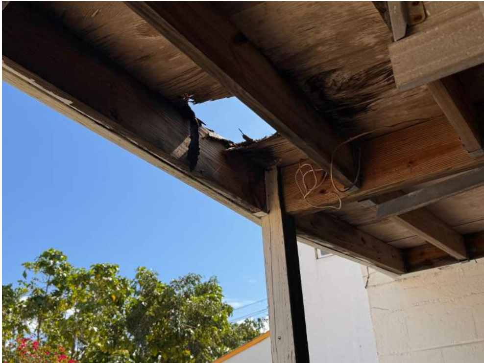
Covered side yard exhibiting failure
