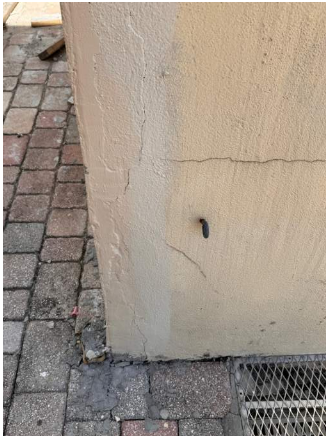
Stucco cracking throughout property
