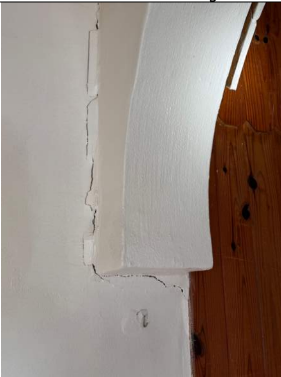
Beam cracking
