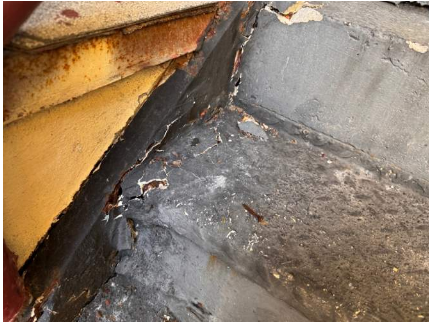
All connections have failed
