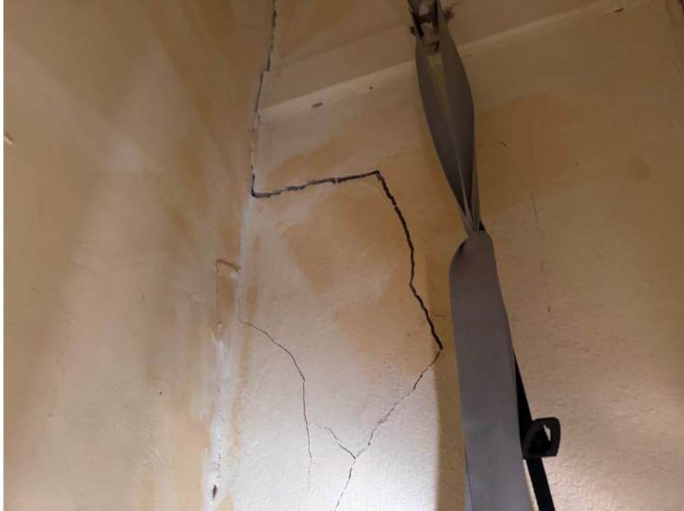
Cracking in the 2 nd floor walls
