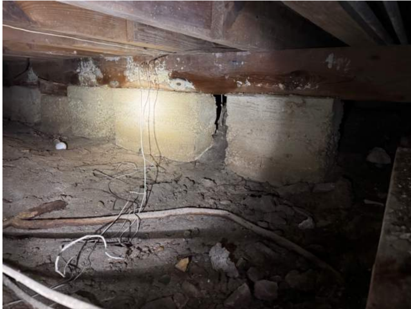
Damaged first floor joists and beams
