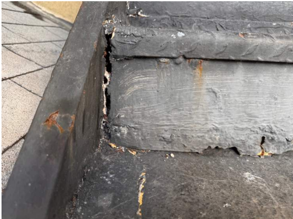
Steel staircase 80% failed
