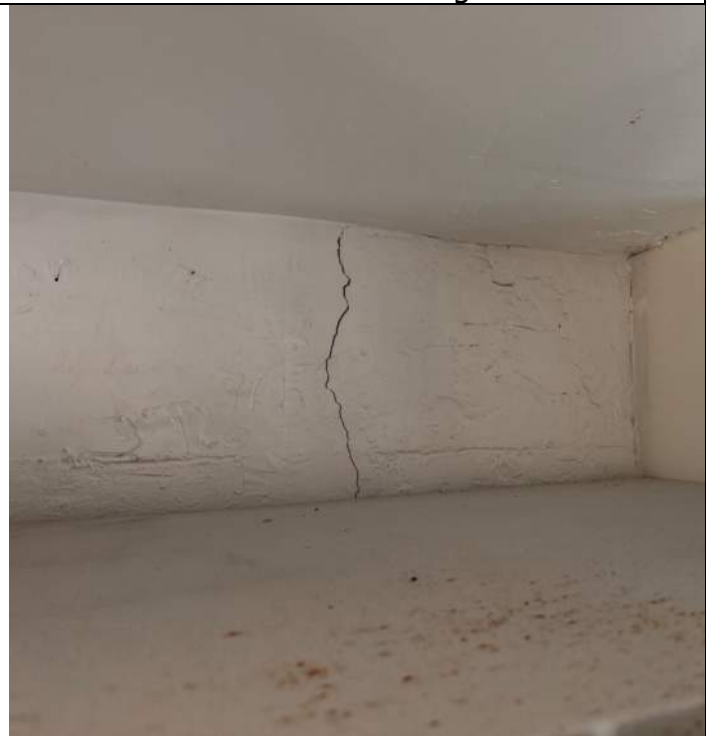
Beam cracking
