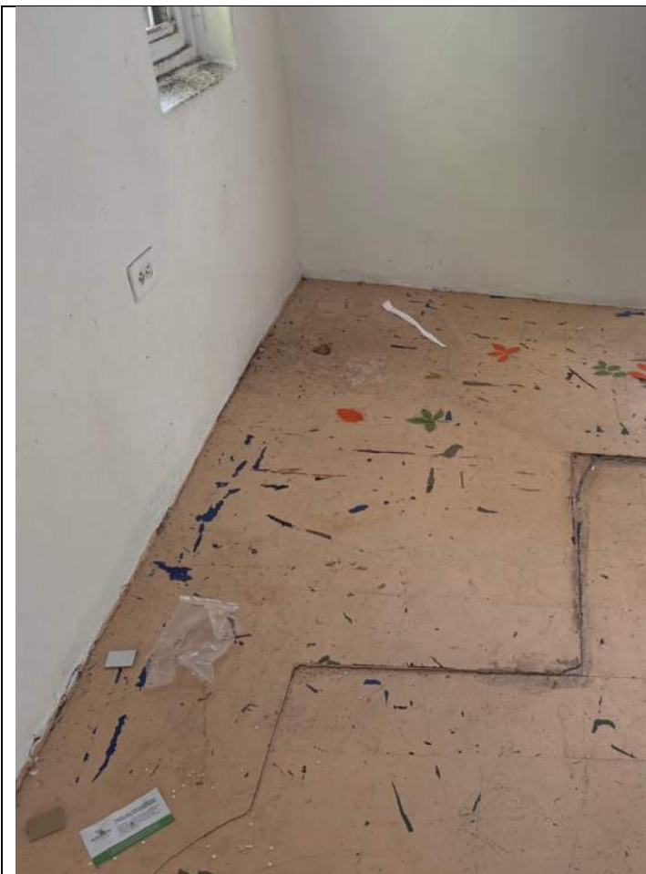
2 nd floor cracking and settlement
