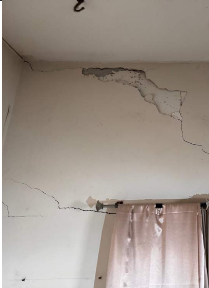
Wall cracking and settlement and leaning towards canal
