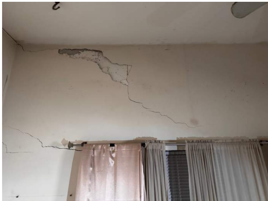
Units 6 walls cracking and evidence of settlement and leaning towards canal
