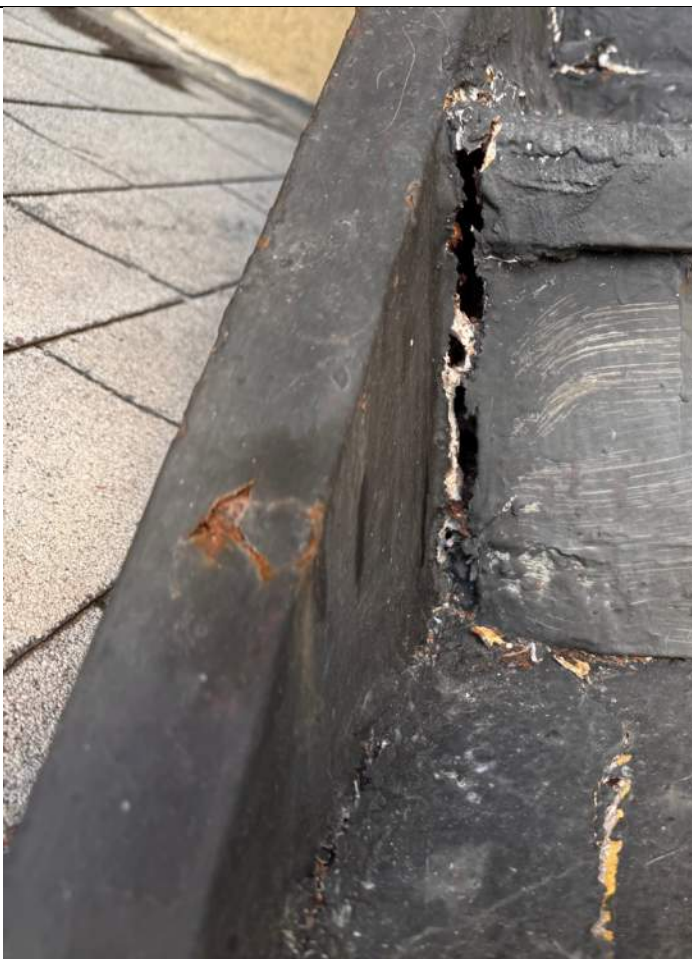
Steel stair connections failure
