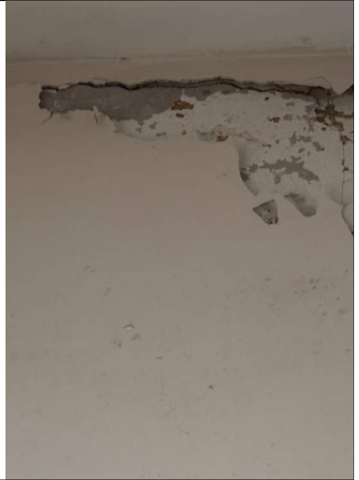
Wall cracking and seperation
