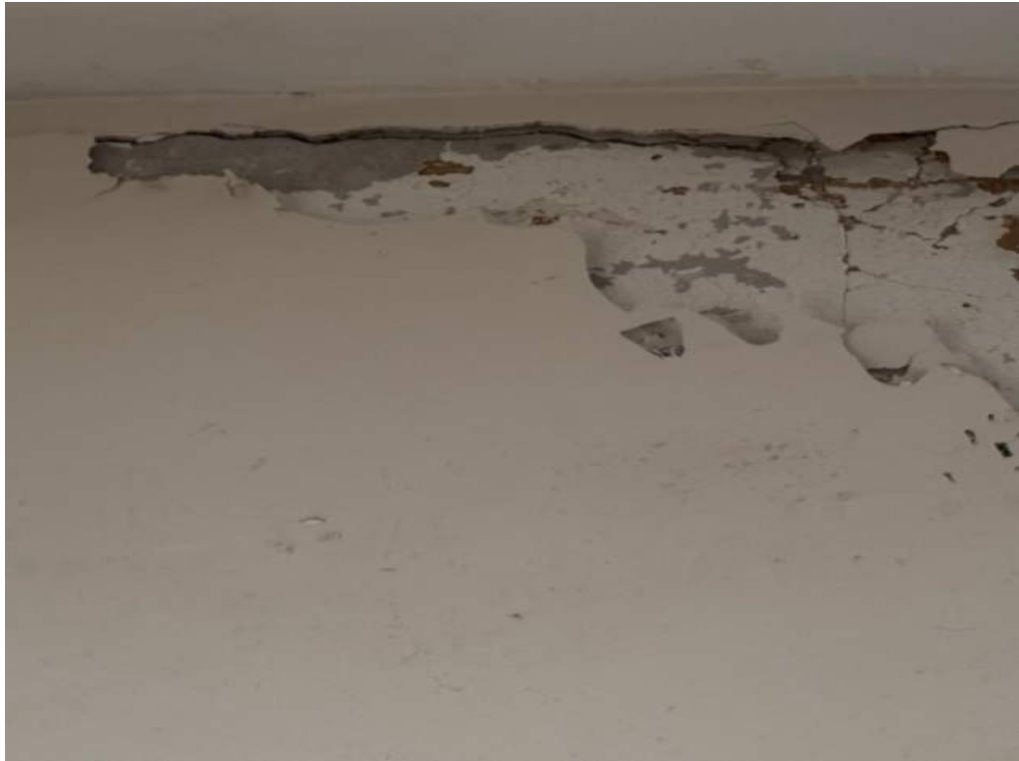
2 nd floor walls cracking
