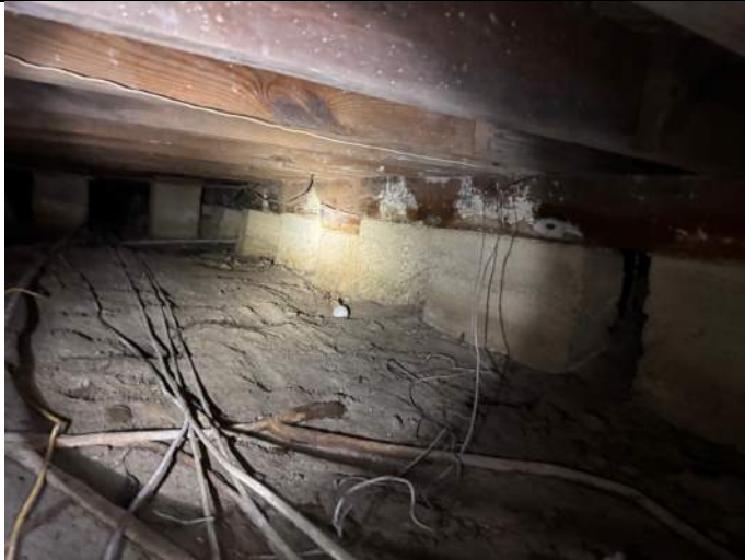
Foundation view showing damaged beams
