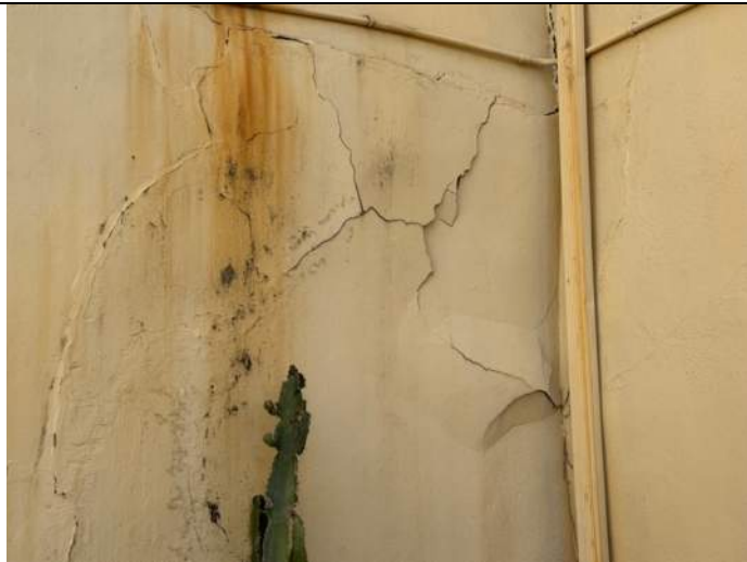
Wall cracking
