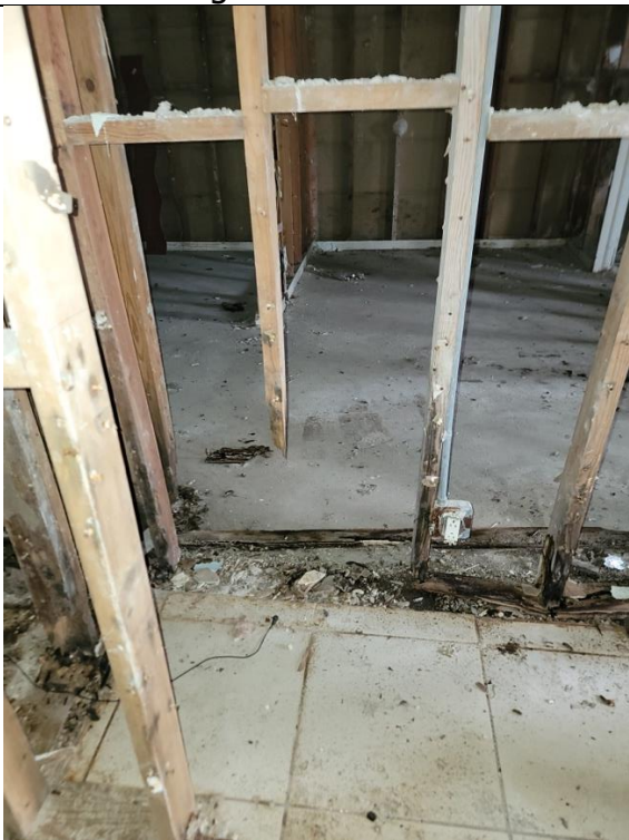
Load bearing stud walls 100% failure
