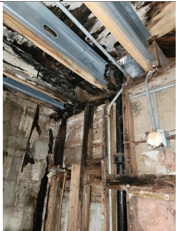
Moisture intrusion damage
