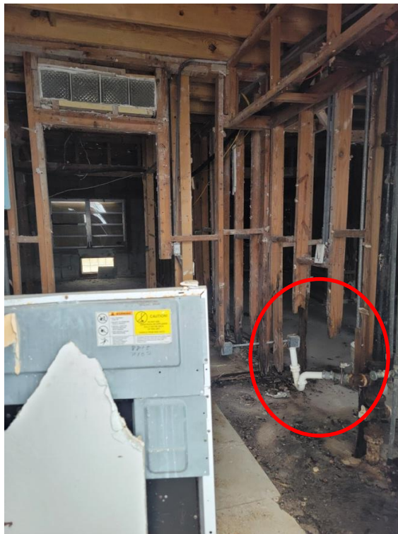
Throughout the building, there is loadbearing wall, stud deterioration, and loss of capacity up to 100%
