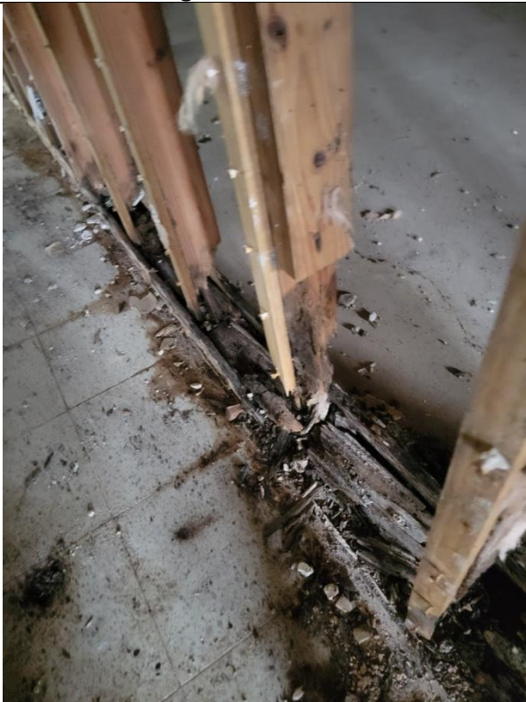
Load bearing stud walls 100% failure
