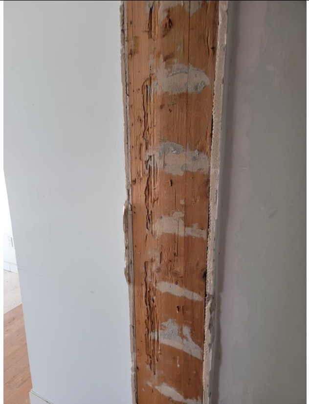
Termite Damage
