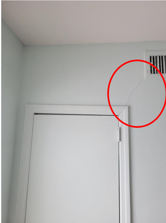
Diagonal cracking of drywall from corners of doors, indicating settlement of foundations
