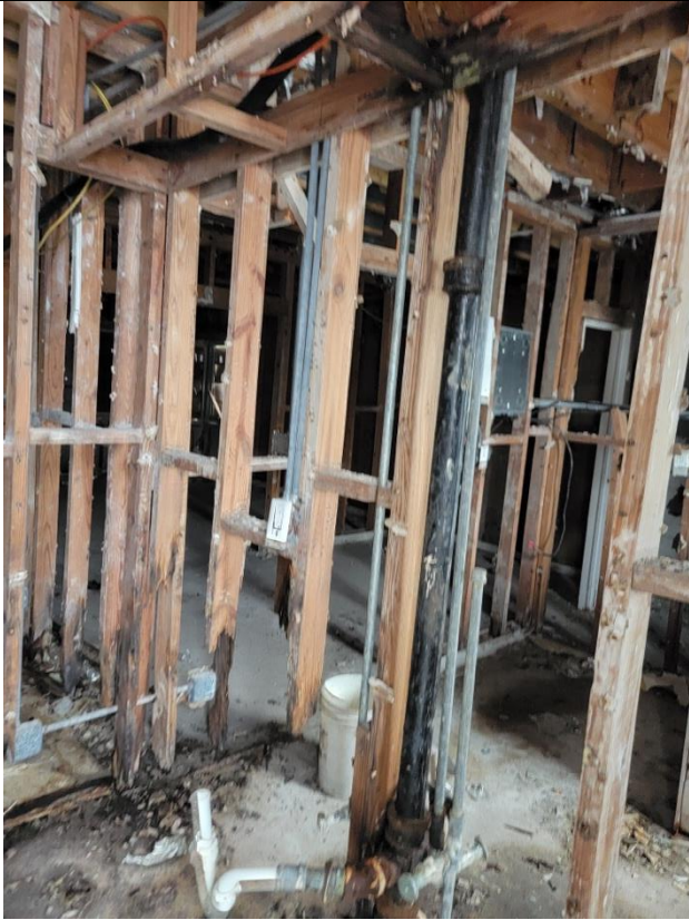
Load bearing stud walls 100% failure
