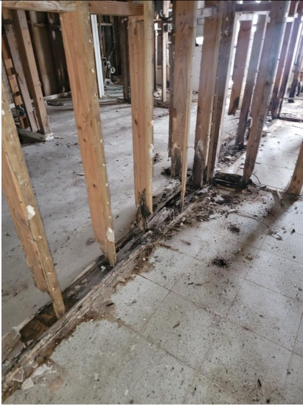
Load bearing stud walls 100% failure
