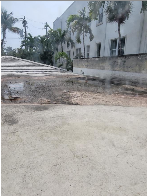
Waterproofing membrane failure
