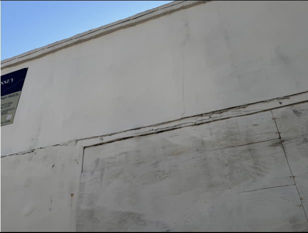
Photo 7 – Exterior stucco with cracks
