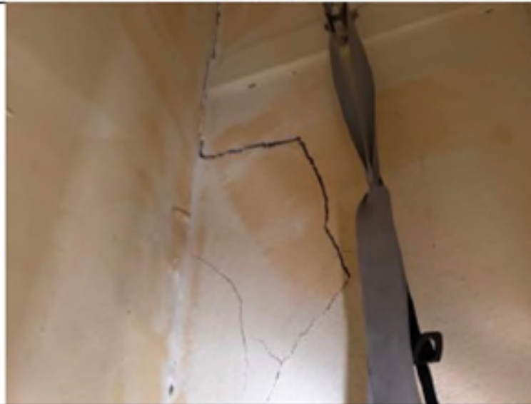
2 nd floor cracking
