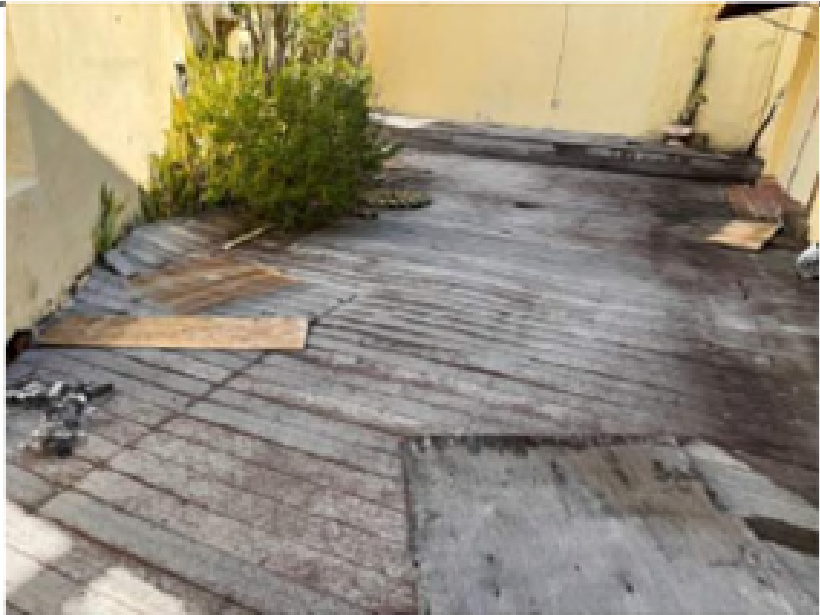
Uneven decking and subfloor failure
