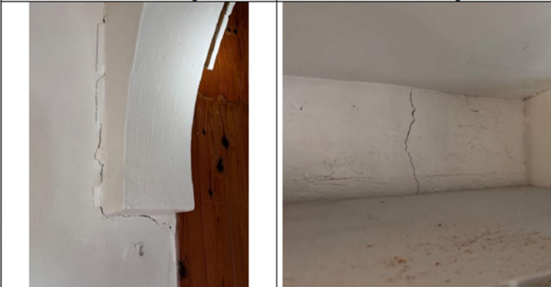
Beam cracking
