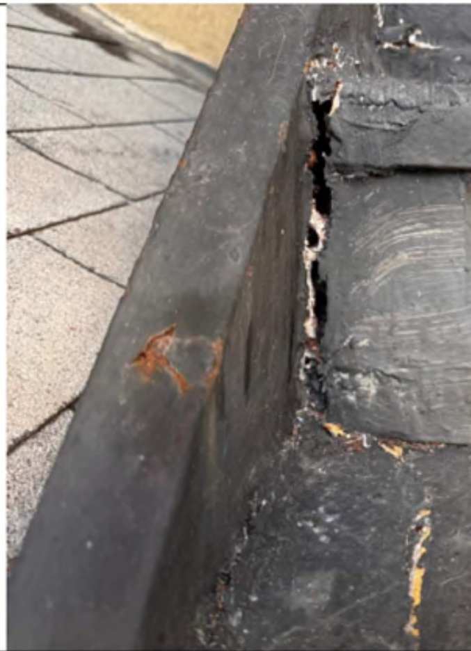
Steel stair connections failure
