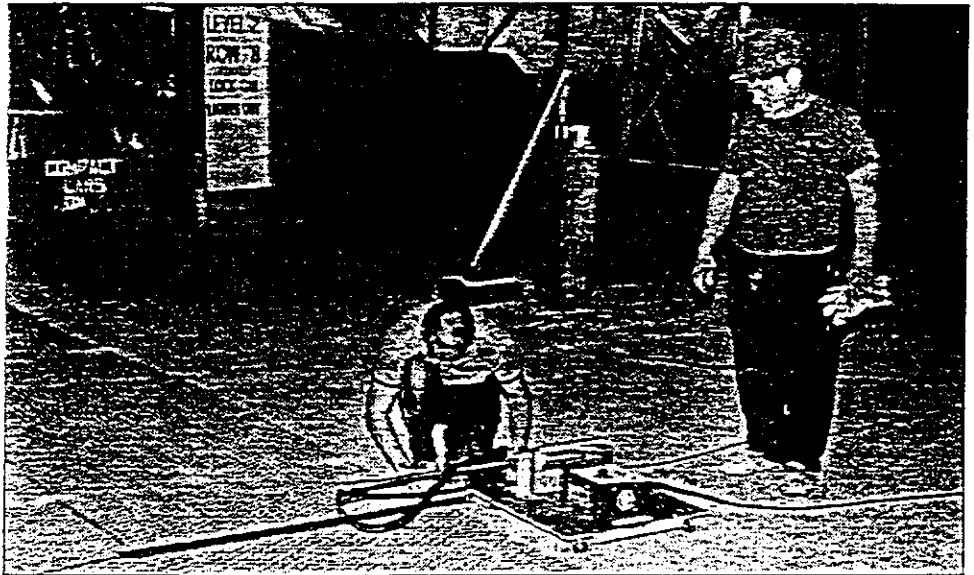
Installing cathodic protection
