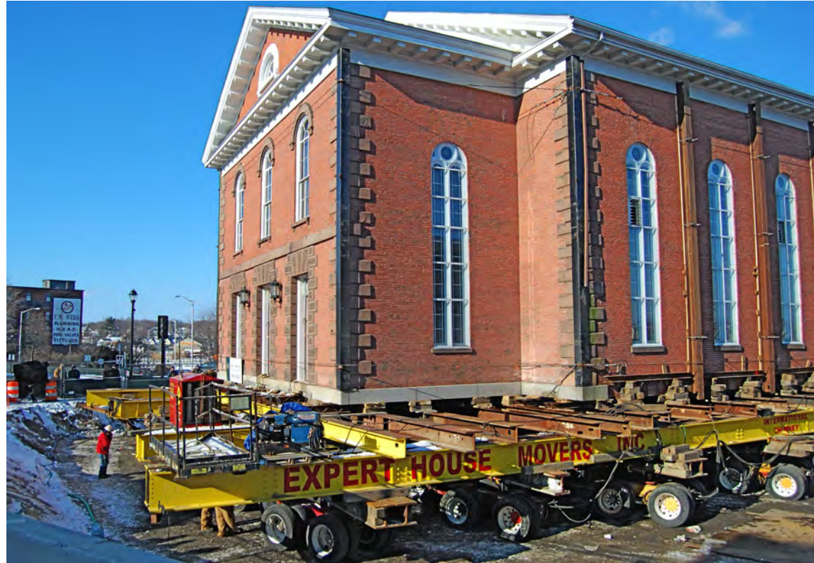
Hydraulically powered dollies move a historic 19th-century brick church in Salem, Massachusetts.
