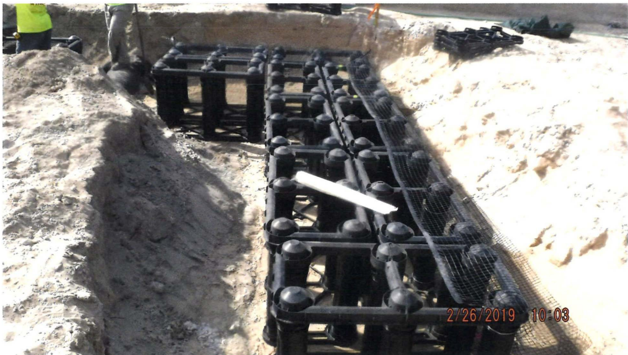
Suspended Pavement System Installation Progress Photo
