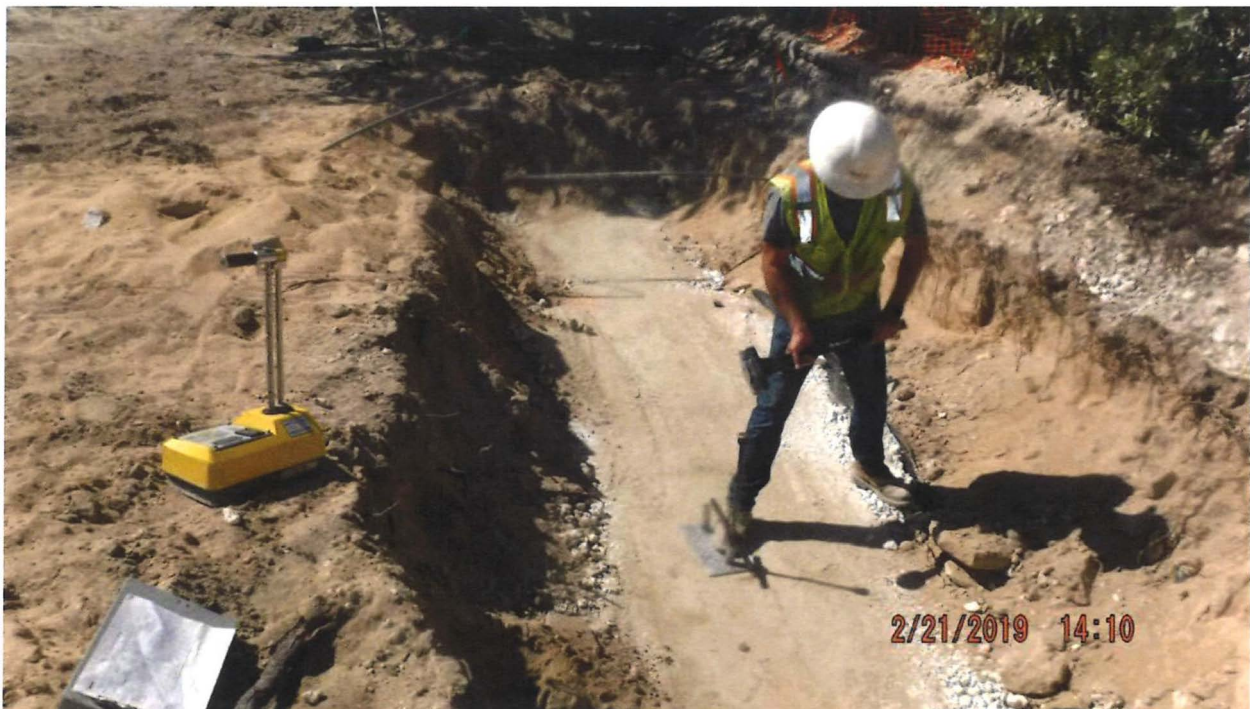
Suspended Pavement System Installation Progress Photo
