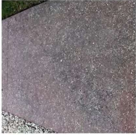
INTEGRAL COLOR RED CONCRETE WITH EXPOSED SHELL AGGREGATE
