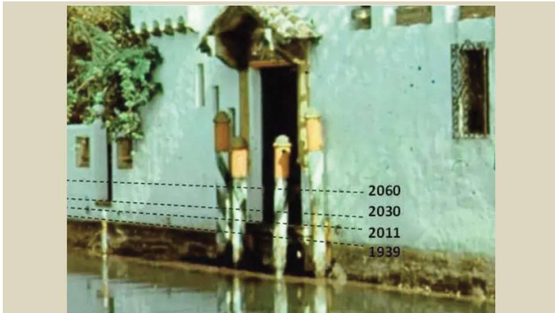
A 1939 photo shows position of the high water mark on the wall of 1818 Michigan Ave, along the Collins Canal. Also shown are the height of the high water mark in 2011 and its expected height in 2030 and 2060.
