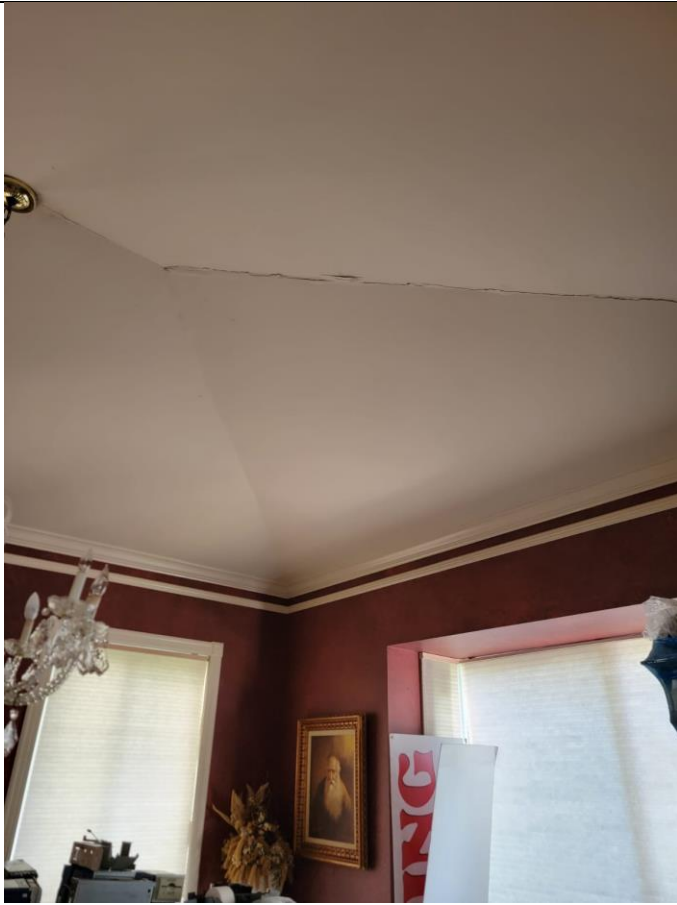
Roof sagging and finish cracking
