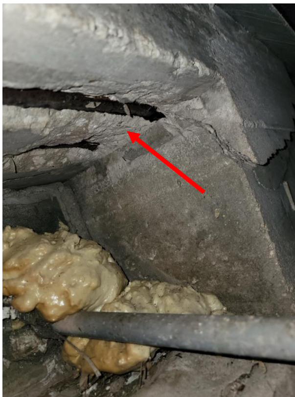
Damaged foundations
