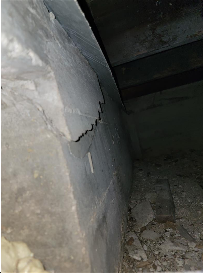
Foundation cracking and spalling
