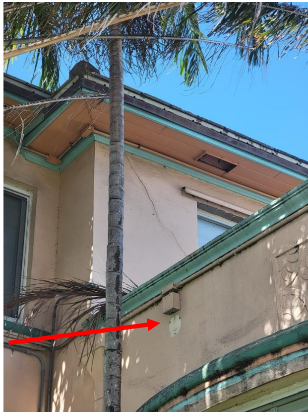
Wall Cracking Due to Settlement
