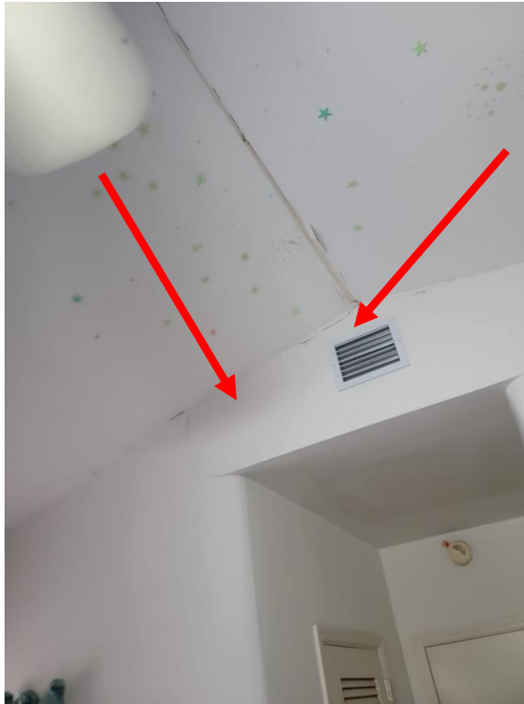
Roof Deflections and moisture intrusion
