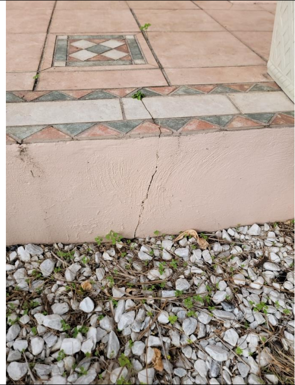
Foundation cracking
