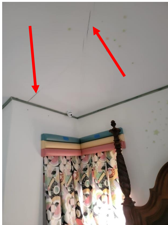
Roof Deflection and moisture intrusion
